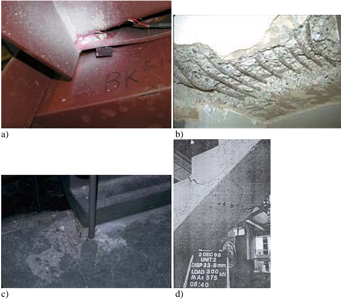
Fig. 8 – Examples of damage state DS2 for stairs: a) Weld cracking on steel stair (photo by C. Higgins), b) spalling of concrete stair (La Union, stair damage, Los Palos Grande District, Caracas, Venezuela, (The Earthquake Engineering Online Archive, Karl V. Steinbrugge Collection: S2170S3558), c) concrete crushing and spalling on upper story stair landing after Anchorage, Alaska earthquake, (The Earthquake Engineering Online Archive, Karl V. Steinbrugge Collection: S2170), d) Concrete crushing, spalling, and significant cracking (Simmons 2000) .
