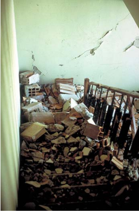
Fig. 3 - Stairway in the Banco Central Building, Managua, Nicaragua (1972 Managua Earthquake). Debris on stairs from the failure of the hollow tile partitions surrounding the stairs (Photo from PEER Godden Collection, No. J94).
