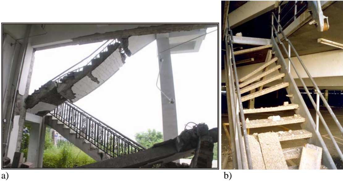
Fig. 9 – Examples of damage state DS3 for stairs; a) Staircase between first and second floors of a two-story RC frame structure building in Dujiangyan, China after 2008 Wenchuan Earthquake. (Photo by Feng Yuan, Earthquake Engineering and Engineering Vibration (2009)), b) Hybrid stairway damaged in 1994 Northridge, California earthquake (FEMA 74, 1994 (image inverted at source location)).
